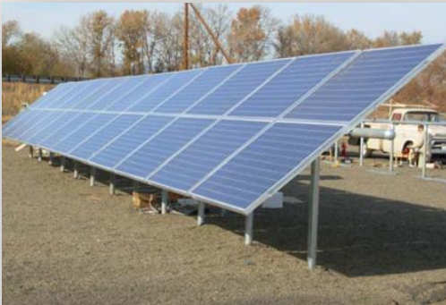
Ellensburg Community Solar
